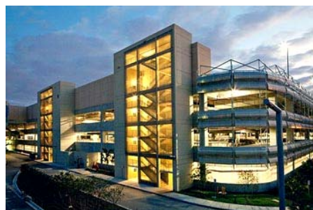
Das neue Rental Car Center RCC
